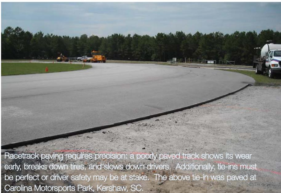
Racetrack paving requires precision: a poorly paved track shows its wear early, breaks down tires, and slows down drivers. Additionally, tie-ins must be perfect or driver safety may be at stake. The above tie-in was paved at Carolina Motorsports Park, Kershaw, SC.
